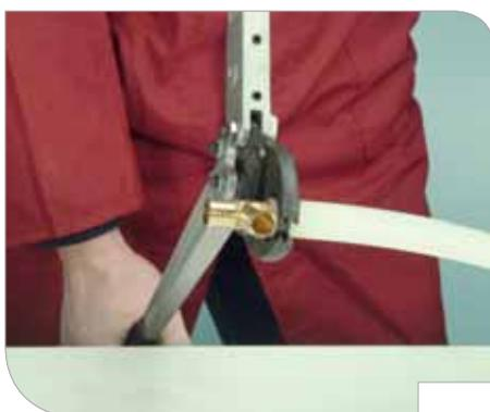
4. Position the tool in a way that the crimp ring is completely covered by the tool jaws. Keep the tool at a 90° angle to the fitting and close it completely.
