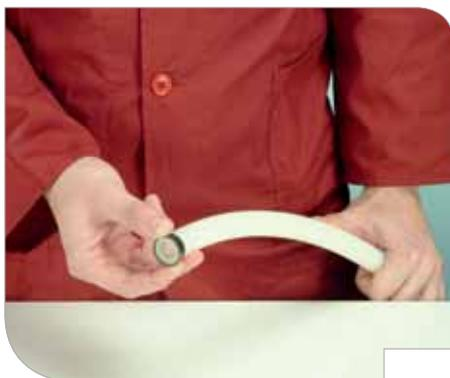
2. Slip the special copper crimp ring onto the pipe.
