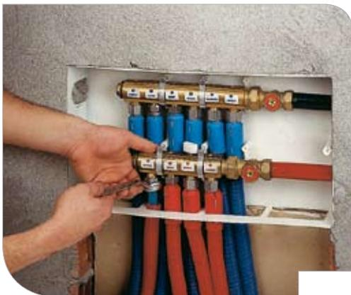
Once the pipe is cut with the right length, proceed with the connection to the manifold. Ends of the pipe are protected with the covers R998.
