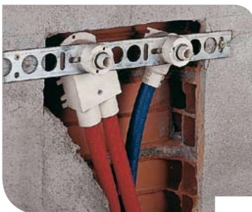
When the assembly is carried out, perform a pressure test, and after that block the fittings and the protection covering of the sleeves with concrete.
