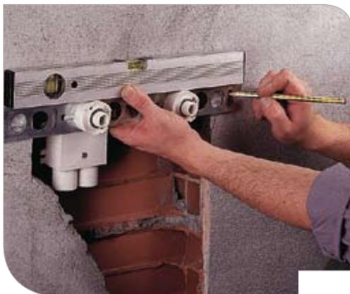
The bar is set to the wall using expansion dowels and a spirit level for the correct position.
