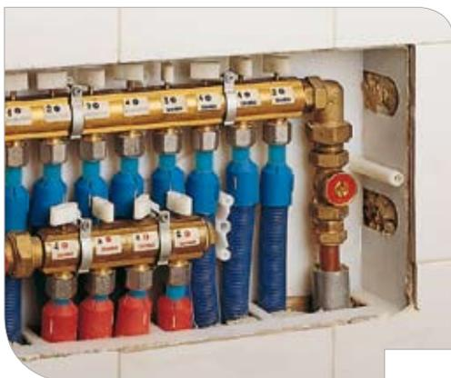
When replacement is over, re-open the lockshield and re-fit the cover of the cabinet.
