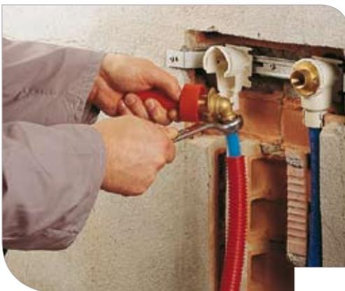
Tightening of the nut of the adaptors is easier when using the end piece R577 and key R131.
