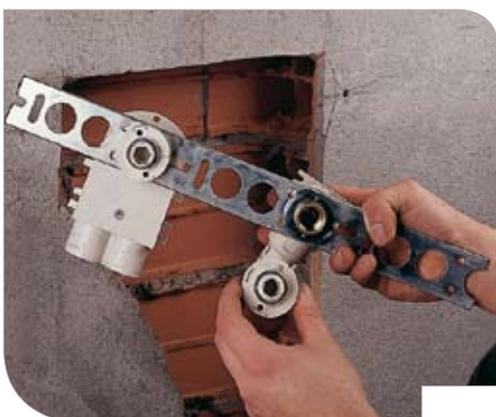
Position the fittings to the bar with the desired interaxis.
