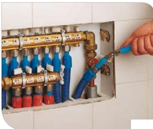
While the pipe is pulled out from the wall fitting side, insert the new pipe on the other side.
