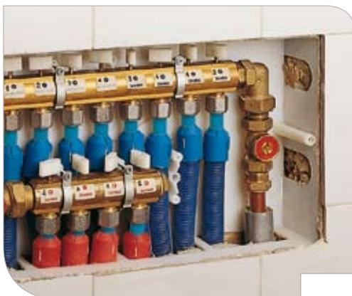
When replacement is over, re-open the lockshield and re-fit the cover of the cabinet.
