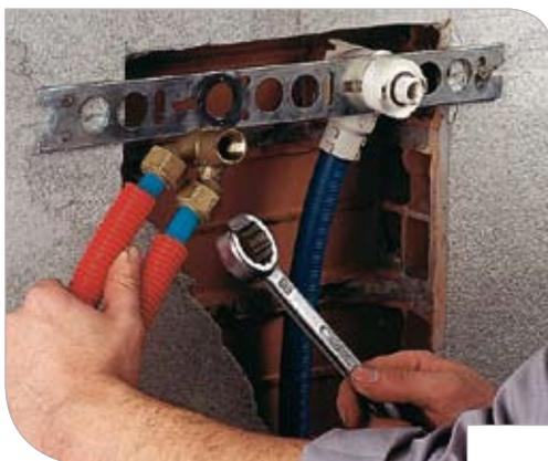
Once the bar is fixed, proceed in connecting the pipes to the fittings.
