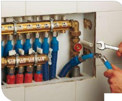
Connect the new pipe to the damaged one with the R576 traction fitting.
