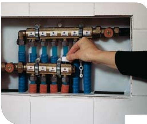
When assembly is carried out, set the single circuits with R73K key.
