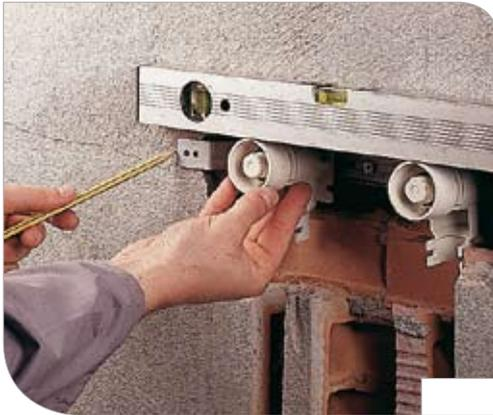
Correct position of the connections is done using a spirit level.
