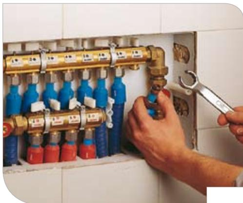
Close the lockshield, untighten the nut of the adaptor and disconnect the pipe to be replaced.
