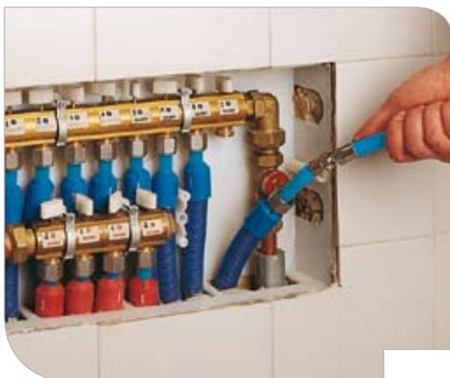
While the pipe is pulled out from the wall fitting side, insert the new pipe on the other side.
