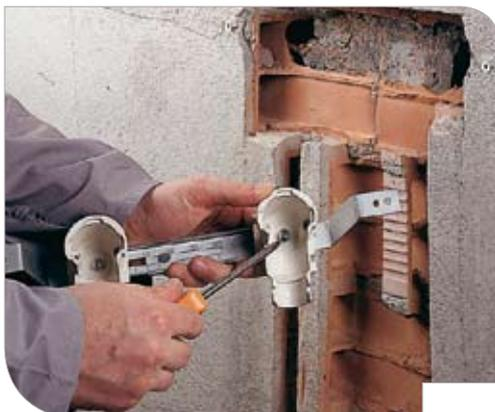
After selecting the required position on the wall for drains and pipes, proceed with the assembly of the fittings using the correct brackets.
